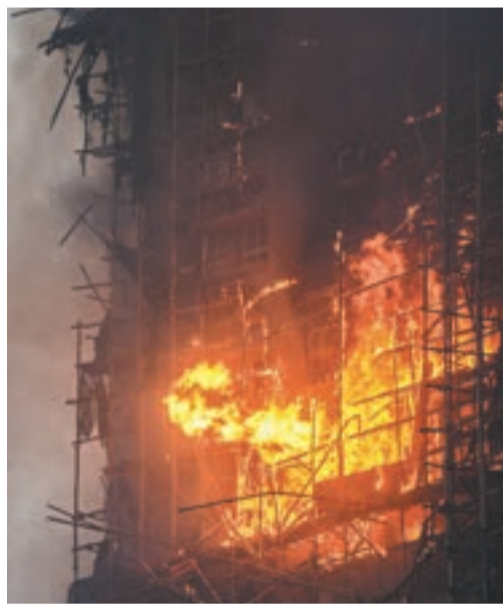
The blaze was intensified by styrofoam, while fire alarms in all blocks malfunctioned. Photo: Eugene Lee
